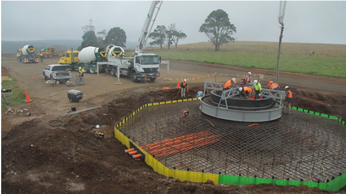
Photograph 5.6: Foundation Construction and Steel Reinforcement 9
