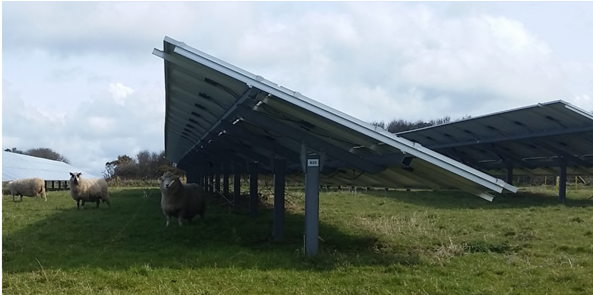
Photograph 5.10: Example of Piled Single-leg Mounting Frame
