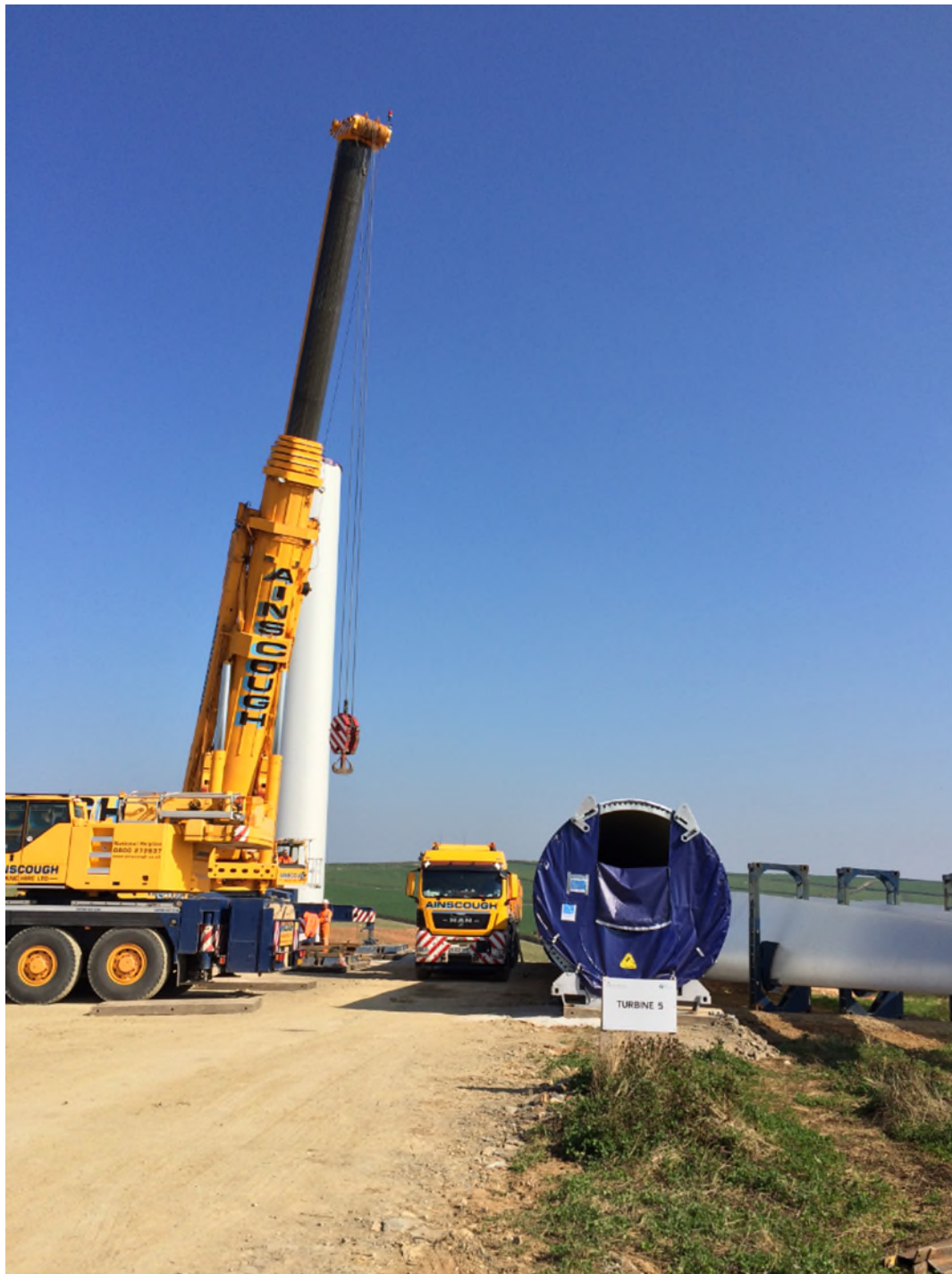
Photograph 5.7: Erection of Tower Sections
