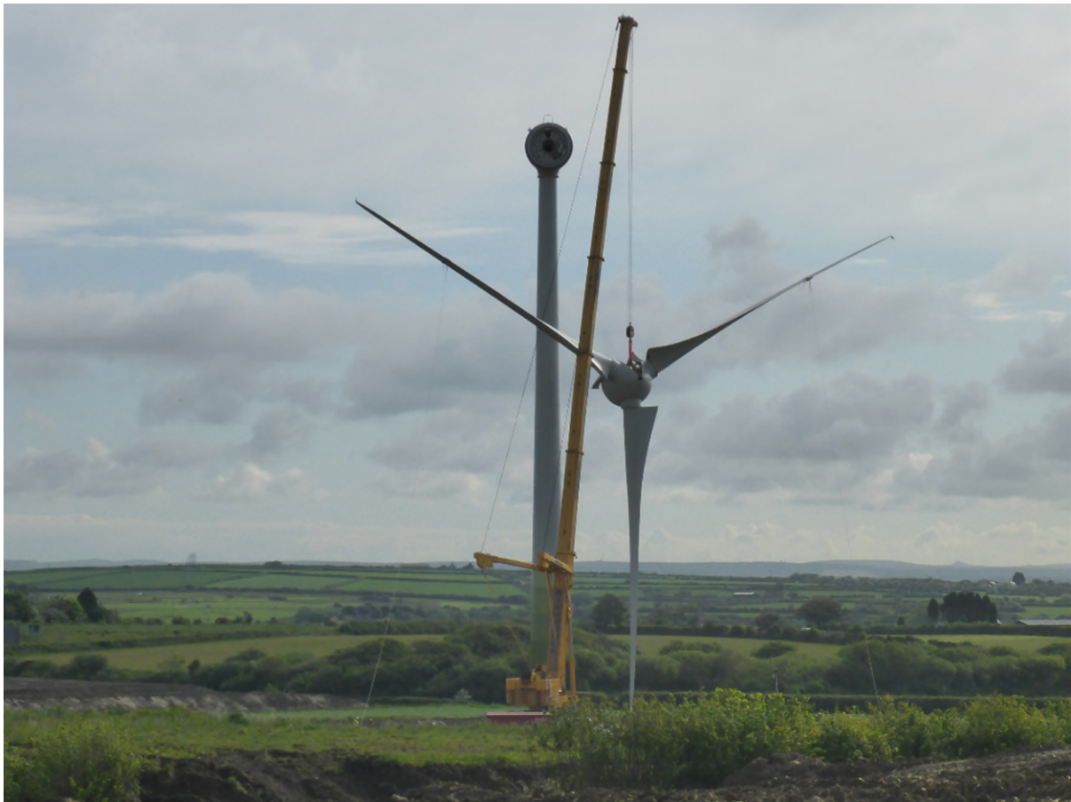
Photograph 5.8: Example of Rotor Lift
