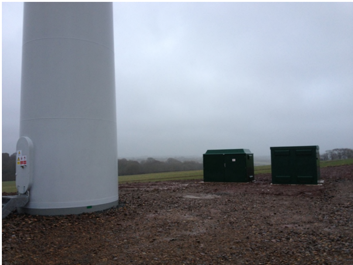
Photograph 5.5: Example of Wind Turbine Electrical Cabinets
