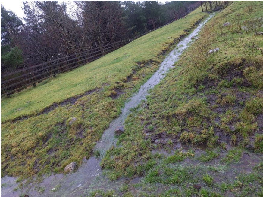
Location: 21 National Grid Reference: SO 10513 08518 Photograph Date: 19/12/2023 Description: On site drainage ditch / field drain. Slightly blocked by vegetation. Concrete culvert where water flows into concrete drainage ditch which flows towards River Rhymney. Flow: smooth, flowing east into culvert. Bottom photo is Location 20 entering Location 21. Channel material: Earth (crumbly) Channel width: 0.5m Channel height: 0.25m Water depth: 0.1m
